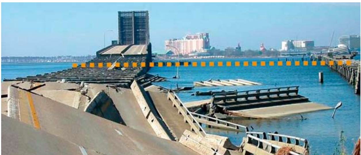
Figure 3 Comparison of deck height on damaged US90 Biloxi Bay Bridge and previously abandoned bridge
